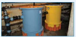
A Solids Separator installed ahead of a Trapzilla® GI servicing the food prep area of a national grocery chain.
